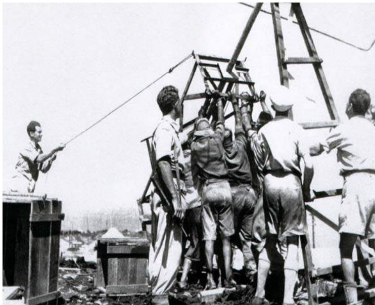
Erecting the antenna for the "homebrew" radar at Haifa. For lack of a suitable electric motor, the antenna was rotated by means of bicycle pedals. (Photo -Maurice Ostroff)
