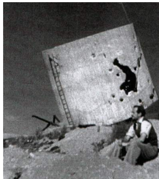
Radar man, Mishy Fine at Yad Mordechai two months after its recapture. The damaged water tower remains a landmark at the Kibbutz to this day. (Photo - Maurice Ostroff)
