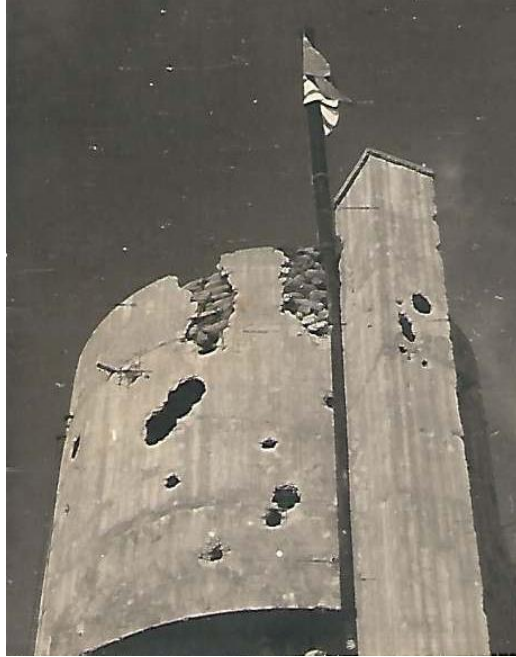
Damaged water tower in Kibbutz Negba
